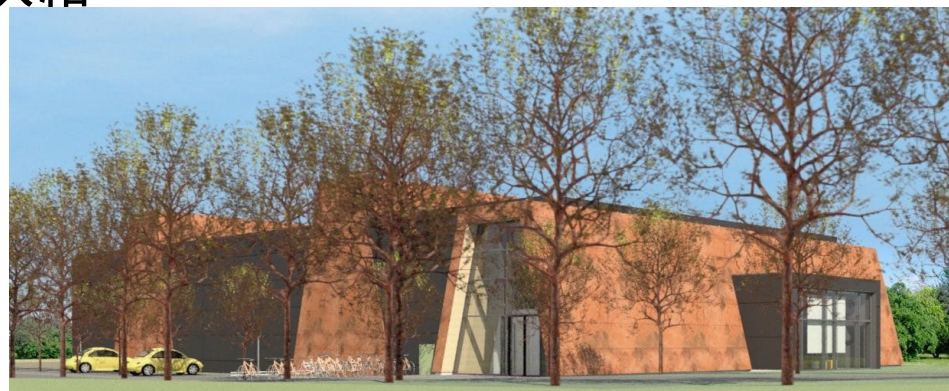
Surplus heat from data centre used for district heating (stateofgreen.com)
